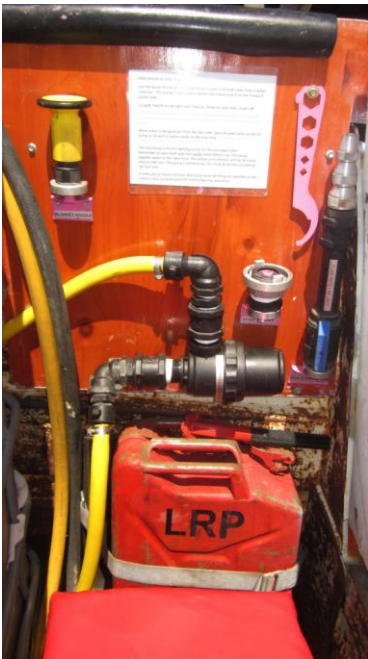
Hose operator station with heat shields ▲ and access to the blanket spray valve
