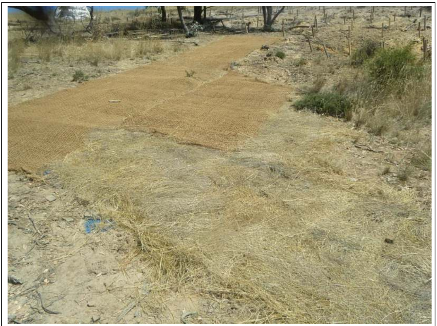
One of the completed matting structures
