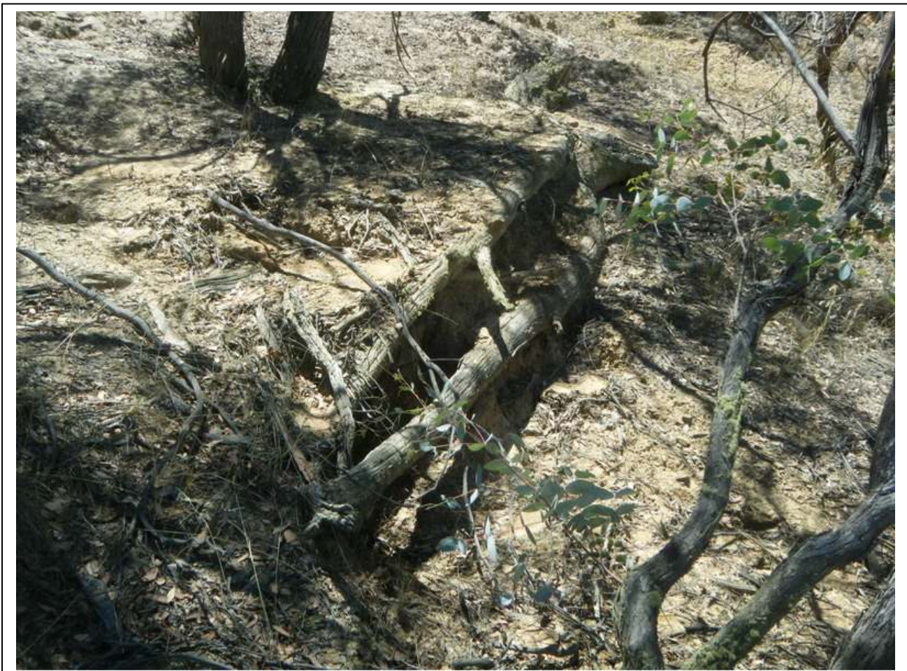
Natural sediment trap on site
