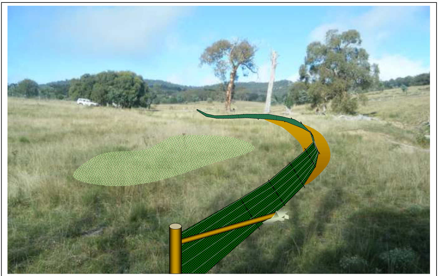
Lower diversion area with bank & restablished grasses. Stage 1.
